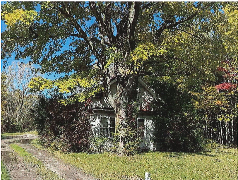
Current Photo from October 2024
